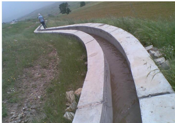
Figure 5. Canal in Xwrmal District [6].
